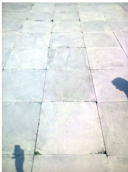
Cement tile with one coat of ThermoDry based emulsion coating
