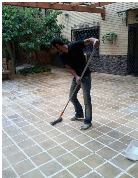
Surface in Niavaran after being cleaned with DeSalin, SurfaPore C and then SurfaShield C were applied
