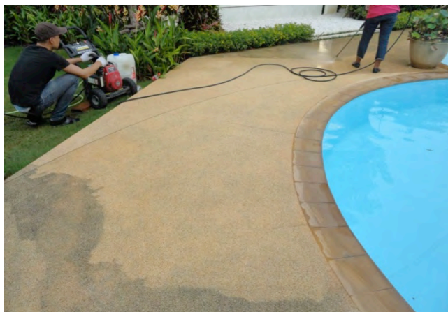
After cleaning with DeSalin K and mold with DeSalin AM, surfaces were treated with SurfaPore C and SurfaShield C
