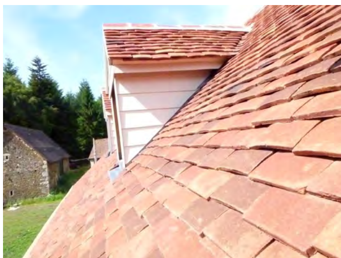
Clay roof tiles 3 years after SurfaPore R treated treatment
