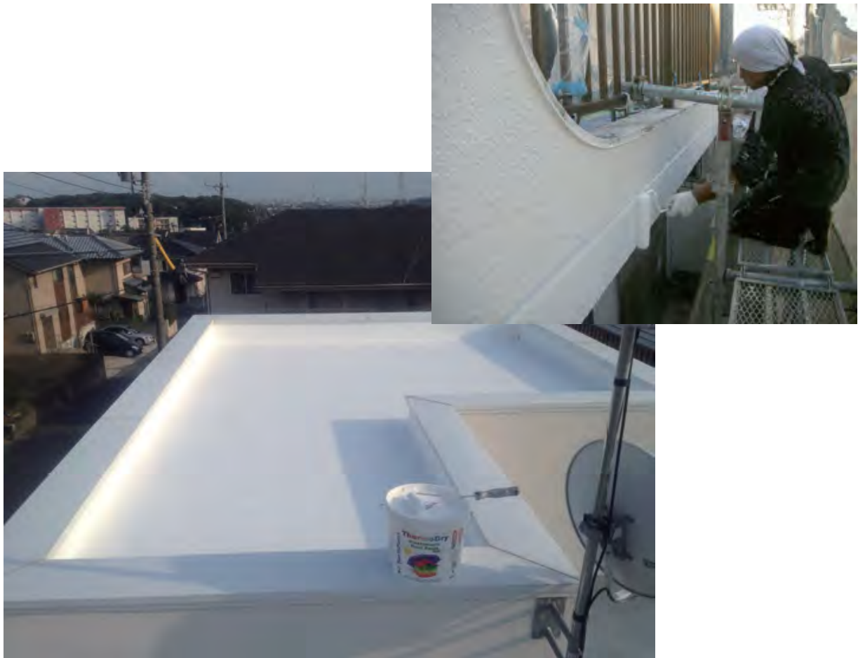
SurfaPaint ThermoDry Elastomeric Roof application
