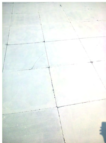
Cement tile with two coats ThermoDry based emulsion coating
