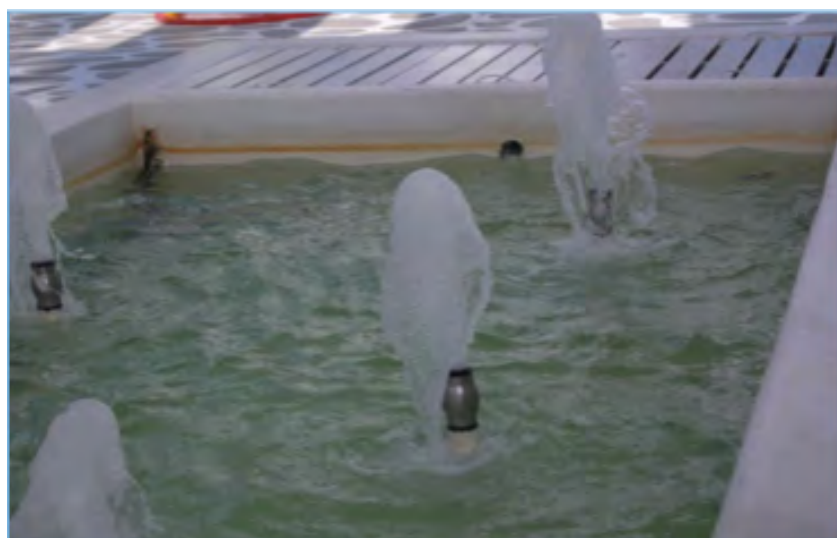
Before SurfaShield C treatment there is evident staining around the pond's edge
